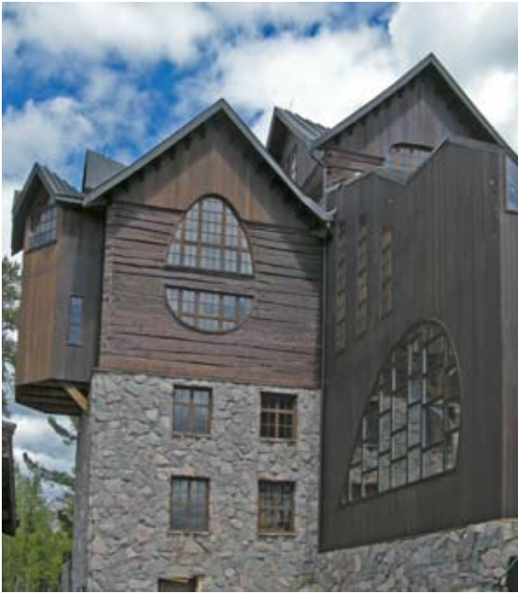
The vision takes shape, including the "Saturn window" at right, designed to mimic the arc of Saturn's rings as seen from a particular angle. That facade features our reclaimed redwood siding, again oiled to bring out a matte, charcoal-colored tone.
