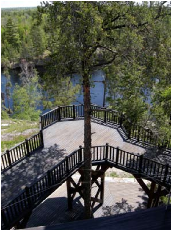
Kemmer (standing left of Steger in the picture here) spent 18 months over three years framing Steger's dream place. The raised walkway through the white pines is all made of our reclaimed redwood. Steger prefers it oiled, which weathers to a soft charcoal grey. Kemmer framed the walkway post structure, including one tricky three-legged tower.
